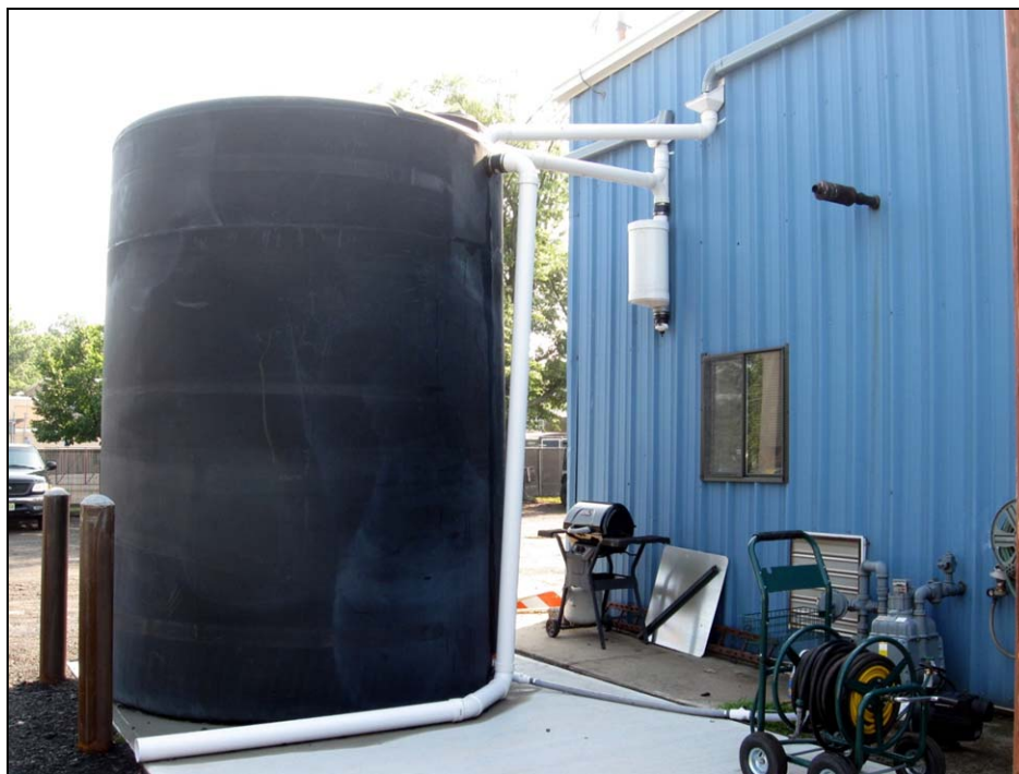
Figure 3. Cistern draining Clark’s Public Works building
