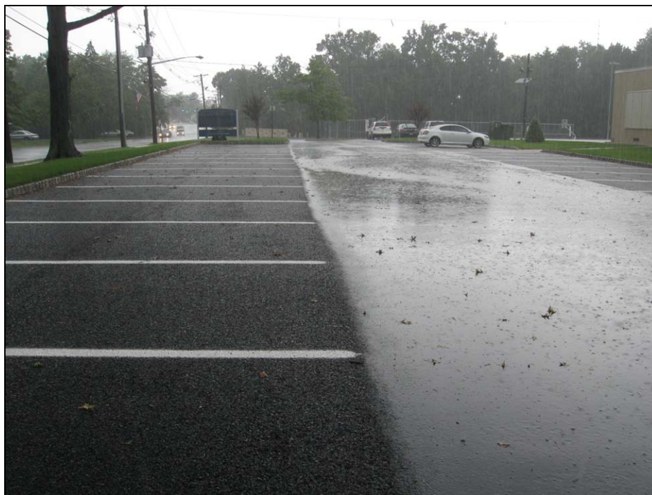
Figure 2. Image shows porous asphalt in parking lanes and conventional asphalt in the driving lane.
